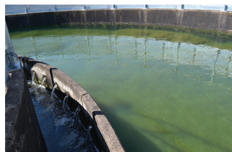
Accelerator with sludge blanket
