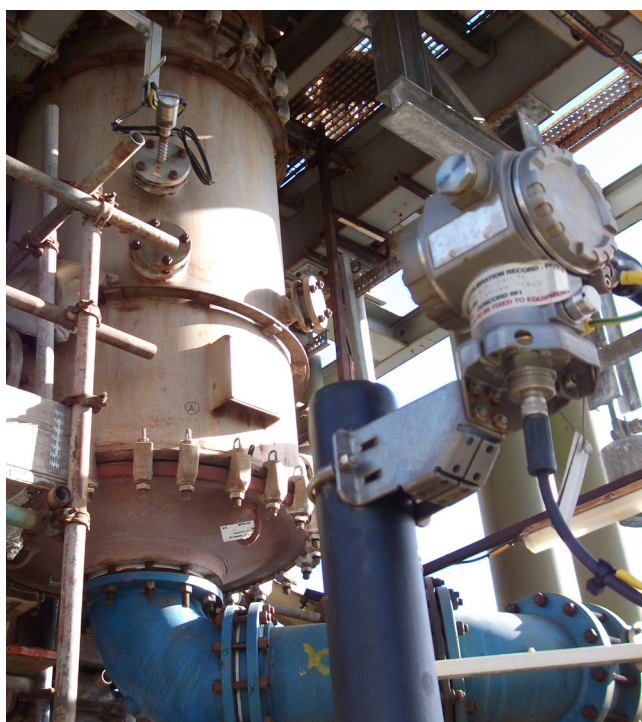
Bottom sensor and separate transmitter.
