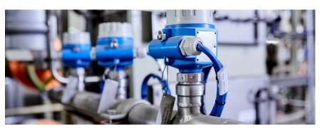
Liquiphant (compact vibration point level switch) used for leakage detection and to protect the hydrogen-cooled generator.
